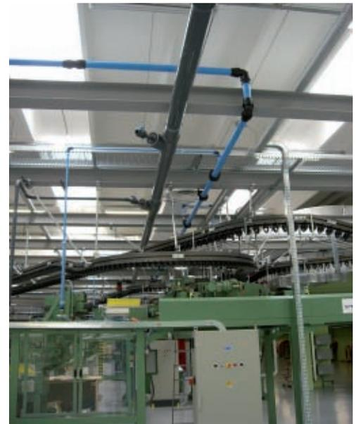
As per the above table AIRCOM pipeline networks have to carry the EC marking only if the network is totally or partially formed by DN 100 pipes and fittings (external diameter 110 mm) and if the maximum allowable pressure in the network is higher than 10 bar.
